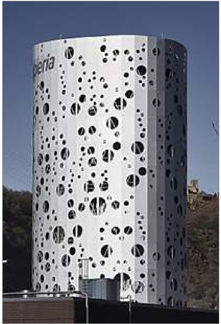
Figure 6 5600 m 3 hot water storage tank in Bolzano, Italy
