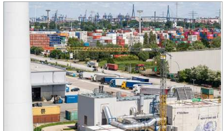
Figure 4 The wind turbine giant Siemens Gamesa has opened a pilot plant for storing electricity in 1,000 tons of volcanic stones. Illustration: Siemens Gamesa.
