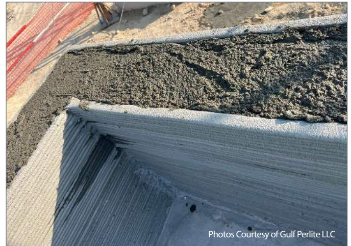
Figure 4 • 3D-printed wall filled with Perlite Lightweight Insulating Concrete.
