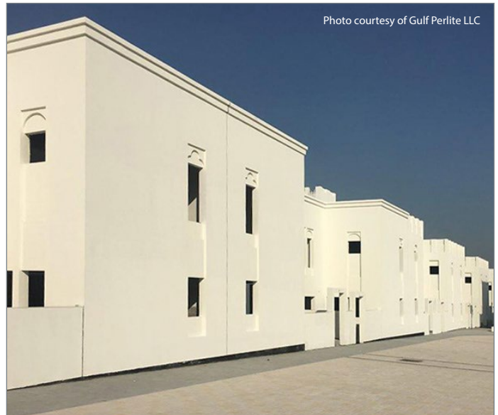
Perlite cement-based lightweight insulating plaster application in a 3,000-unit residential villa project.
