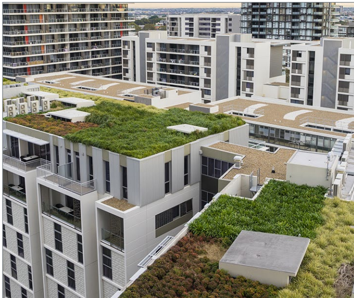
Green roofs made with perlite help manage stormwater, reduce heat island effect, and restore habitat.
