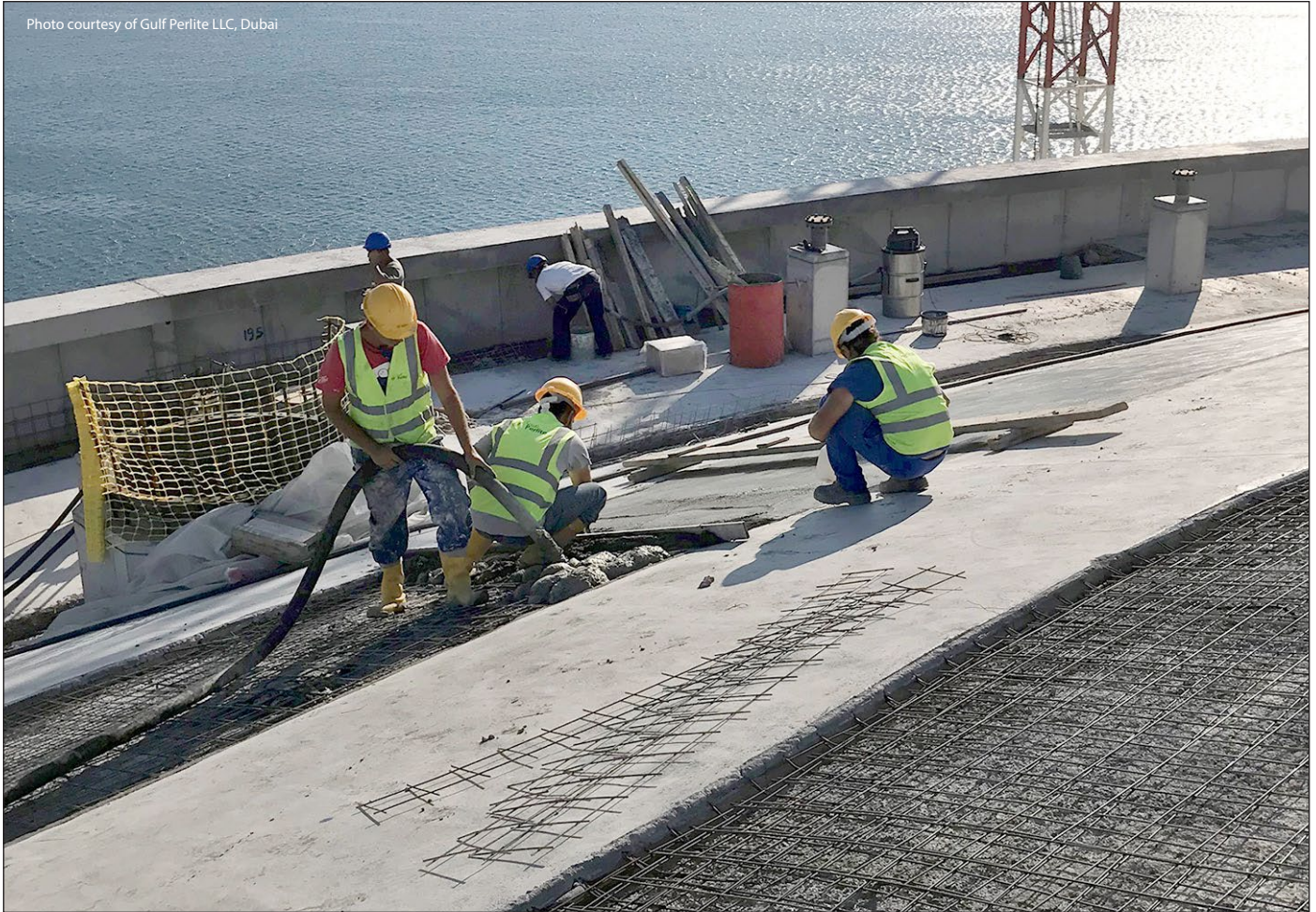
Perlite lightweight concrete forms the roof of this liquefied natural gas (LNG) storage tank
