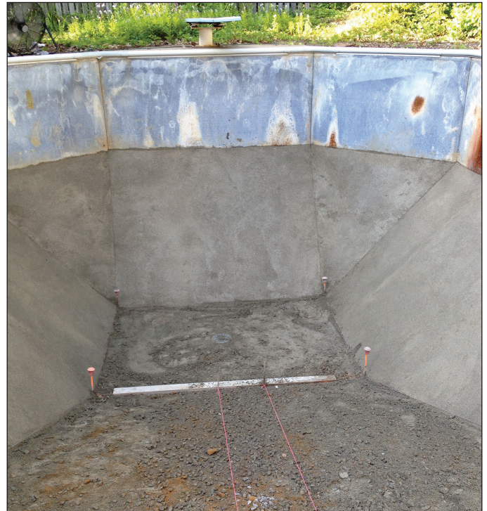
Refurbishing an in-ground pool with a new, insulating, perlite-concrete pool bottom.
