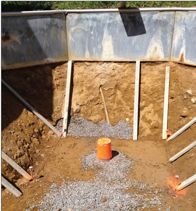
Refurbishing an in-ground pool with a new, insulating, perlite-concrete pool bottom.
