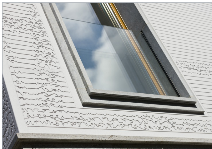
Above: An exterior siding panel using perlite as the filler.
